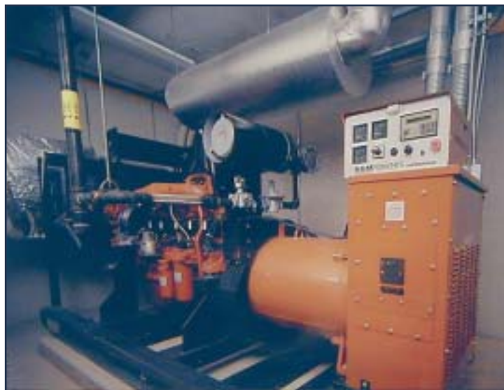
A 1,000-KW natural gas-fired emergency generator
