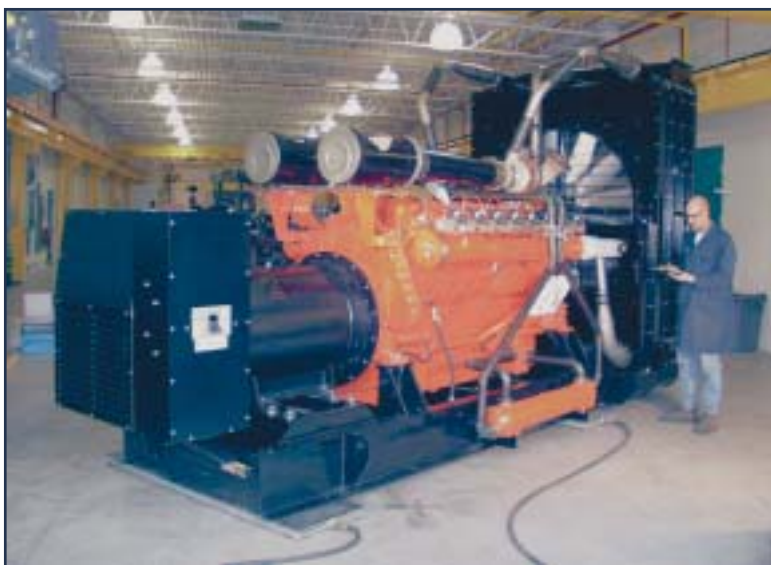
A 1,000-KW natural gas-fired emergency generator
